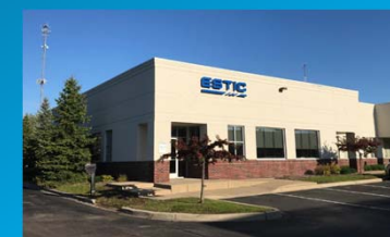
Novi Technical Center
