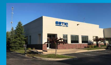
Novi Technical Center
